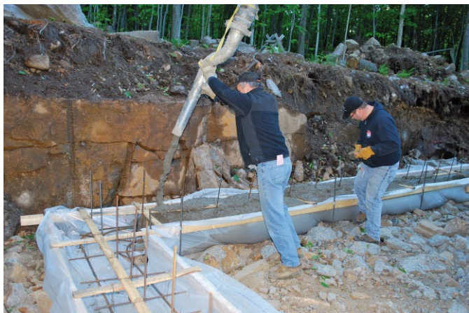
Fig. 7. Fabric-formed strip footing; photo: Fab-Form [25]
