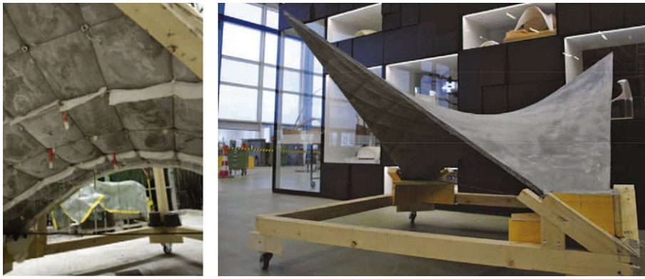
Fig. 12. Hybrid cable-net and fabric-formed shell; photo: Block Research Group, ETH Zurich [45]
