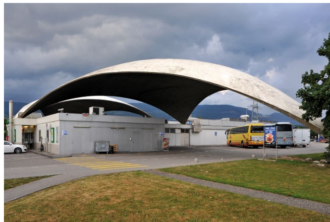
Fig. 9. Reinforced concrete canopy by Heinz Isler; photo reproduced under CC-BY-SA/© Chriusha (архива) [88]
