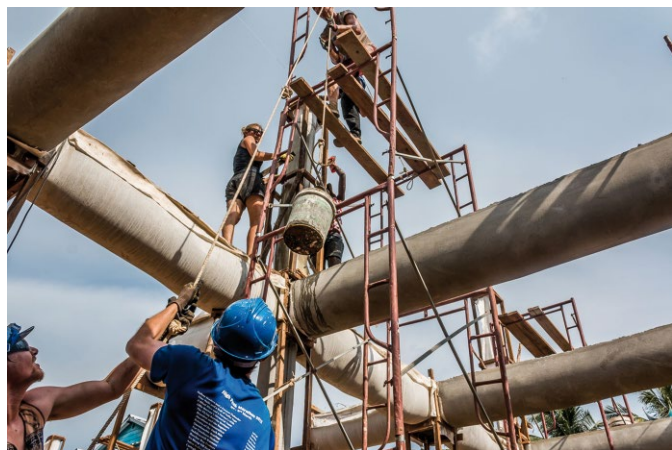
Fig. 4. Fabric-formed beams and columns; photo: Lindsay Perth
