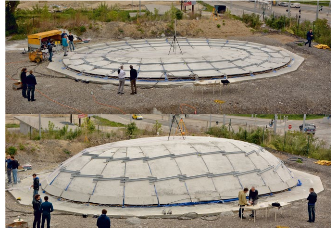
Fig. 16. Pneumatic forming of hardened concrete; photo: TU Wien
