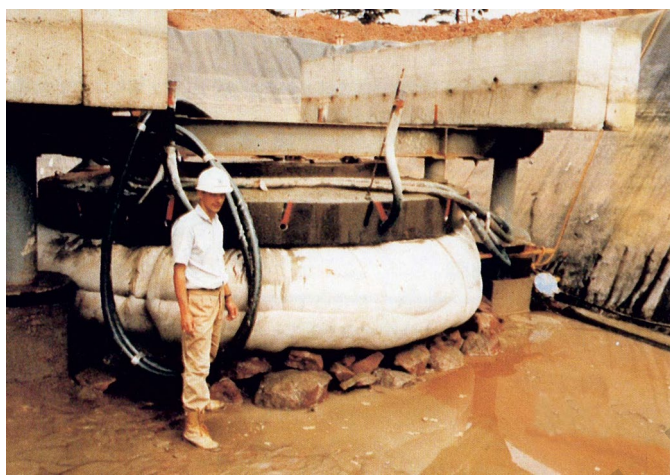
Fig. 8. Footing for a precast marine structure; photo: Proserve Ltd. [84]
