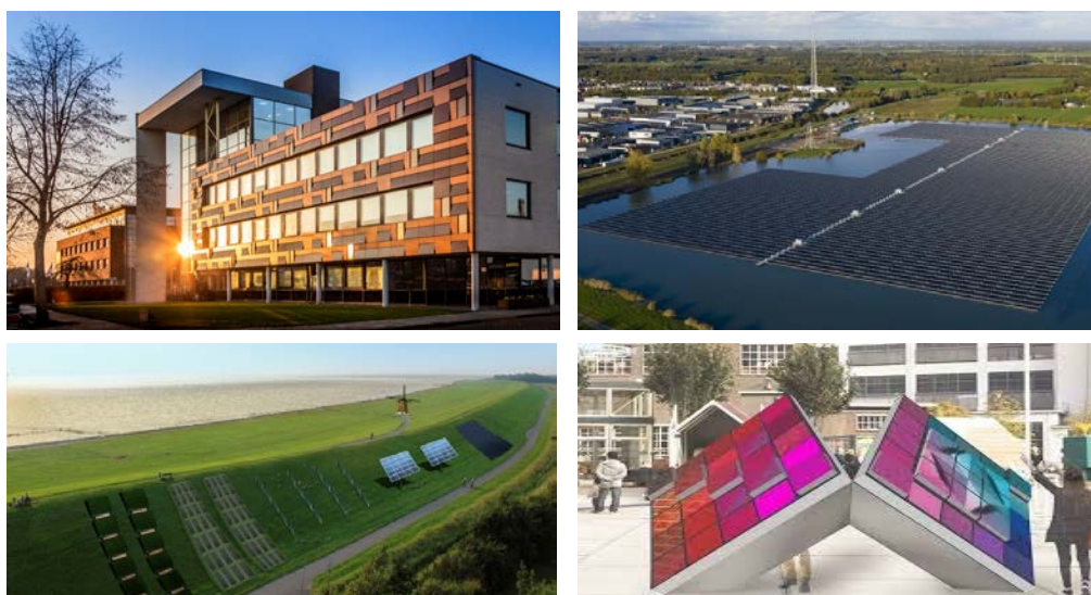
Figure 1: Top left: Kuijpers building Helmond (Netherlands) realized by Kuijpers, Studio Solarix, Sorba and Kameleon Solar; top right: floating PV system realized in 2019 at Sekdoornse plas by GroenLeven and BayWa; bottom left: PV systems applied to slopes of dikes (source: Folkerts), bottom right: innovative colourful design of a PV system in an urban environment (TNO)
