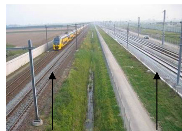
1500 V d.c. 2 x 25 kV a.c. Figure 1a: 1500V d.c. track next 2x25kV a.c. track
