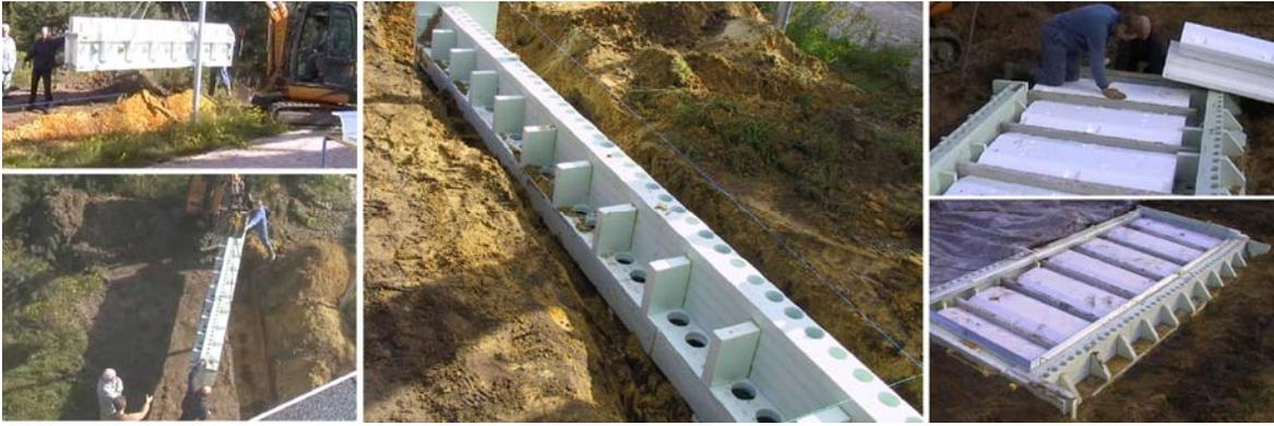
**Figure 4: impression of placing prefabricated elements and floor elements in the pilot project**
