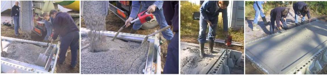
**Figure 5: pouring concrete mortar on ground floor to fill foundation beams of pilot project**
