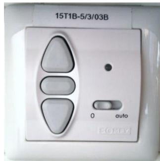
Figure 9. Somfy blinds UI: the switch on the right toggles between automatic and manual modes, while the up/down arrows on the left open and close blinds, move them up and down and the middle button stops the moving blinds.
