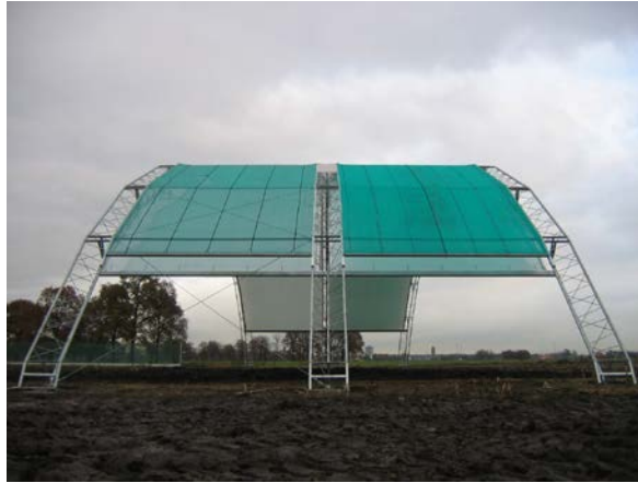
Figure 1.5 Impression of the construction of the arched stable
