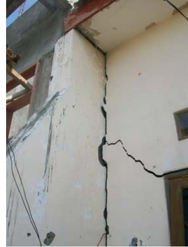
Cracks on the wall influenced by the unstable land condition that caused foundation movement.
