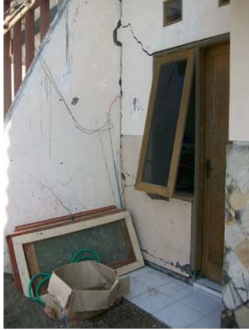
Cracks on the wall influenced by the unstable land condition that caused foundation movement.
