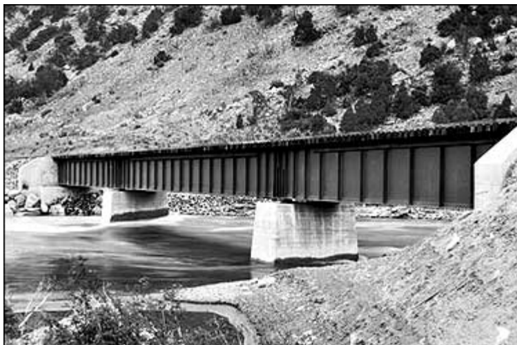
figure 4: flanges applied to prevent local buckling effects
