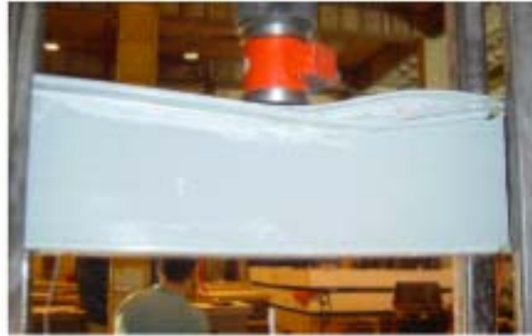
figure 3: flange buckling of an I-shaped beam, a local buckling effect
