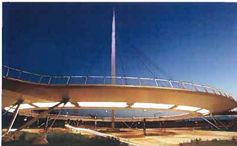
Fig. 1: Cable-stayed bicycle roundabout flyover 'Hovenring' (photo courtesy of Municipality of Eindhoven)
