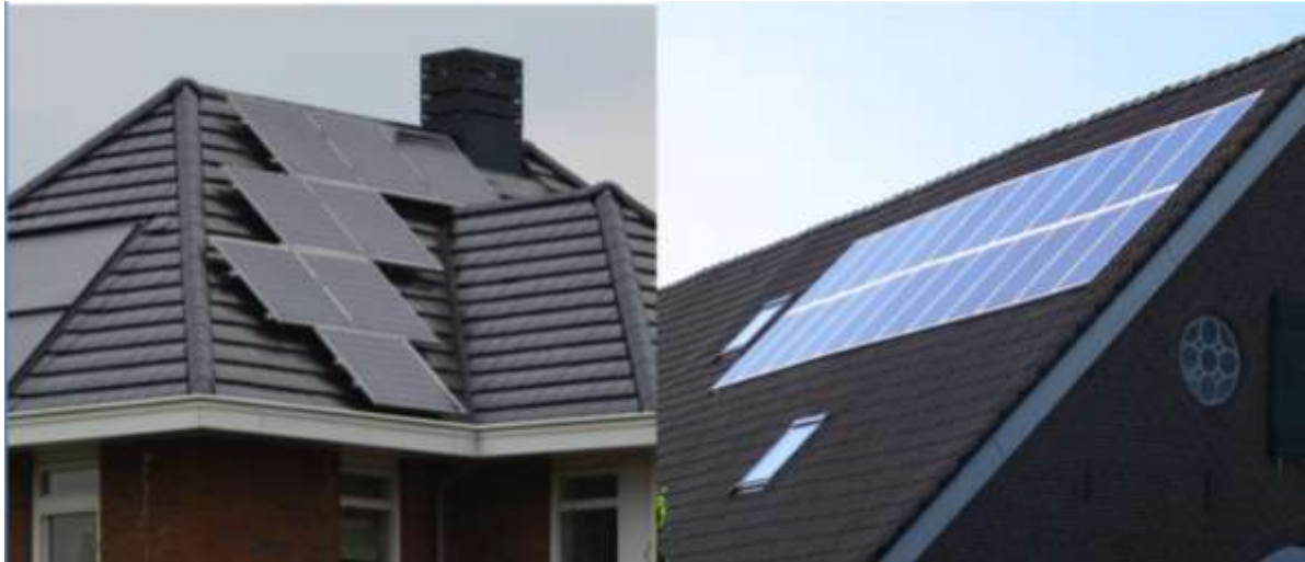
Fig. 1. and 2. Examples of two projects with Building Applied PV (BAPV) and Building Integrated PV (BIPV) in the Netherlands.
