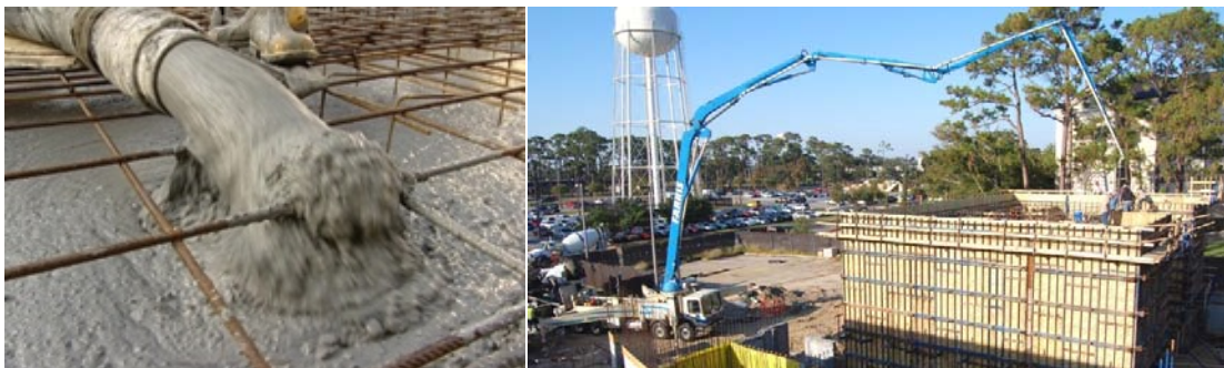
Figure 8: Importance of the pumping ability and travel distance of a concrete mixture
