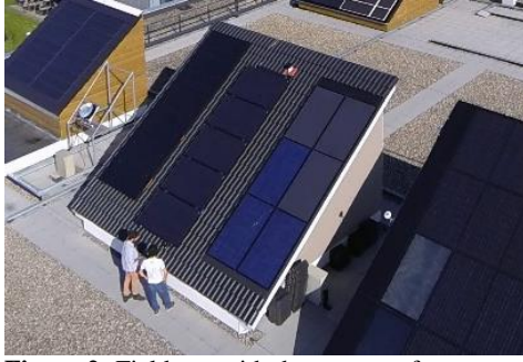
Figure 2: Field test with three types of uncovered PVT systems on the dummy roof in the middle
