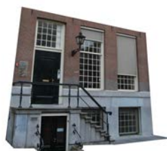
b. cellar – merchant house
